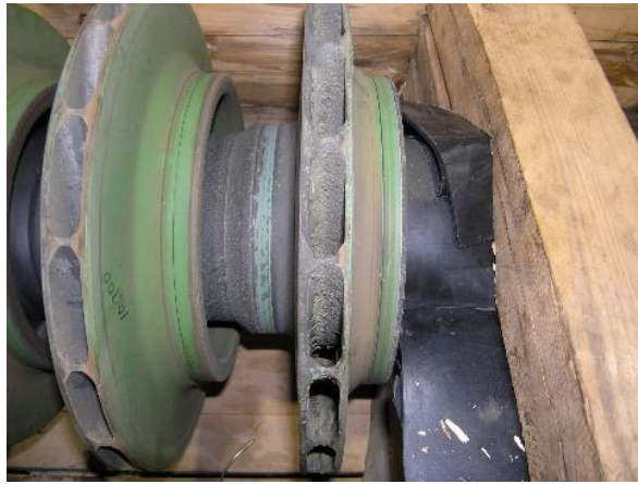
Figure #1. Fouling on impellers. Overnight a large amount of rust peeled off the inlet piping and was ingested causing this fouling and sudden drop in compressor efficiency.
